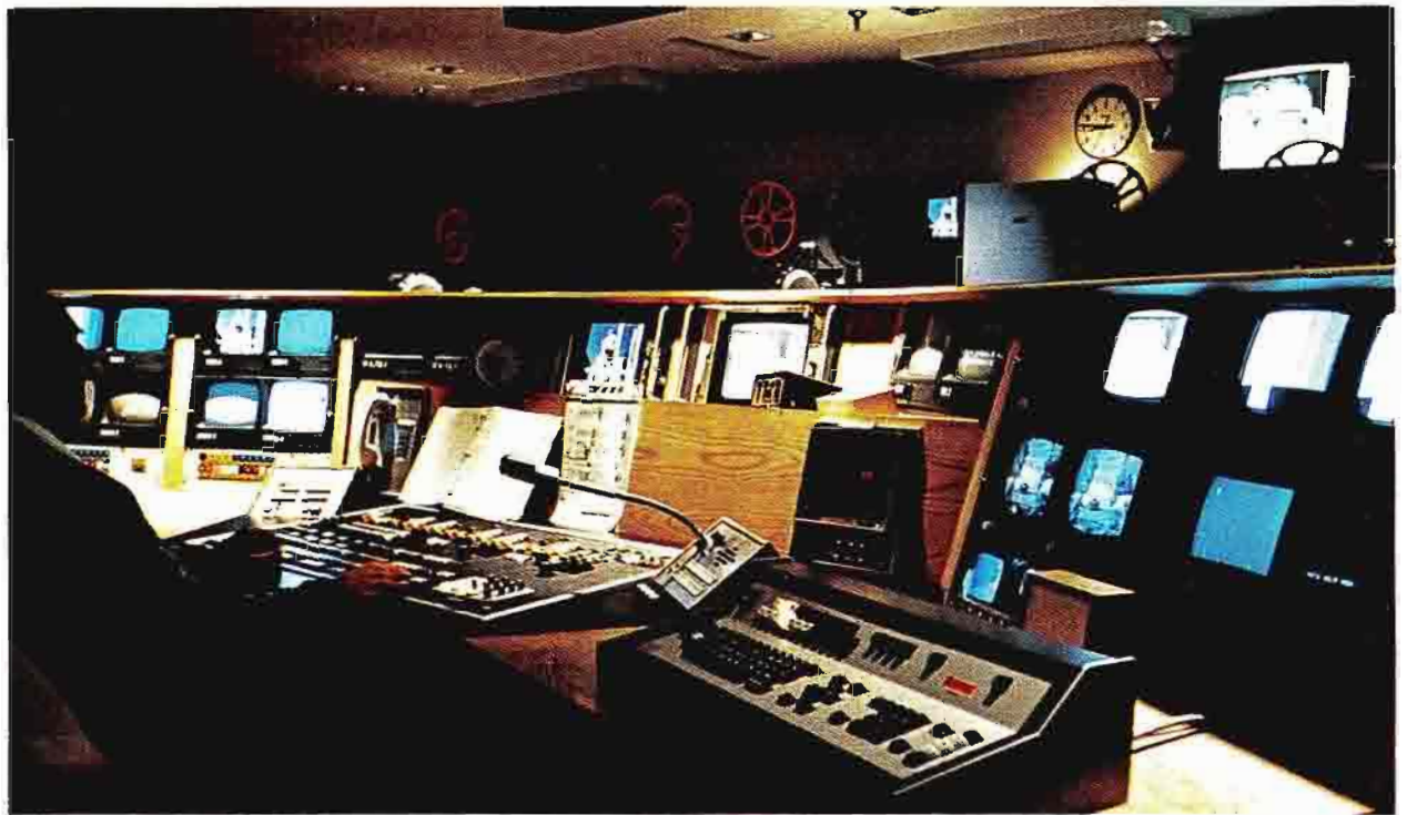
Master Control operator at TV-11 has direct visual contact with four film islands in front of console, and with the adjoining video tape room.
